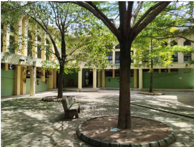
Figure 3.4: View of SMIT complex's biggest courtyard
