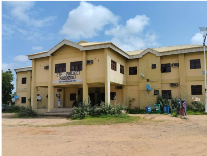
Figure 3.2: Exterior view of the SMIT complex
