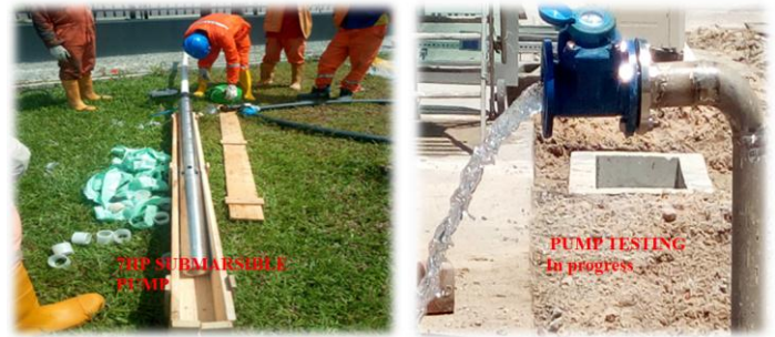
Figure 3: Pumping test in progress at the study area
