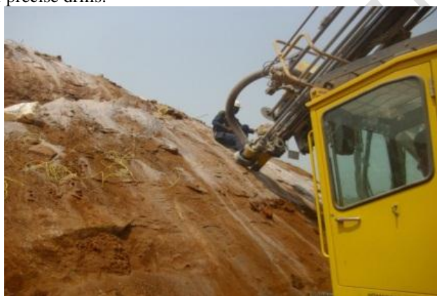
Figure 4: Photo showing drilling in the quarry of Razel-Cam Source: Field work (2013)
