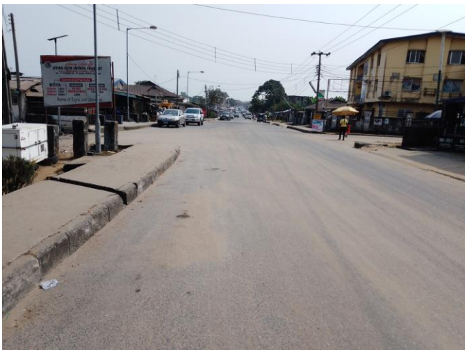
Plate 4: Edgerly Road (Rehabilitated Road with inadequate Street Lights)
