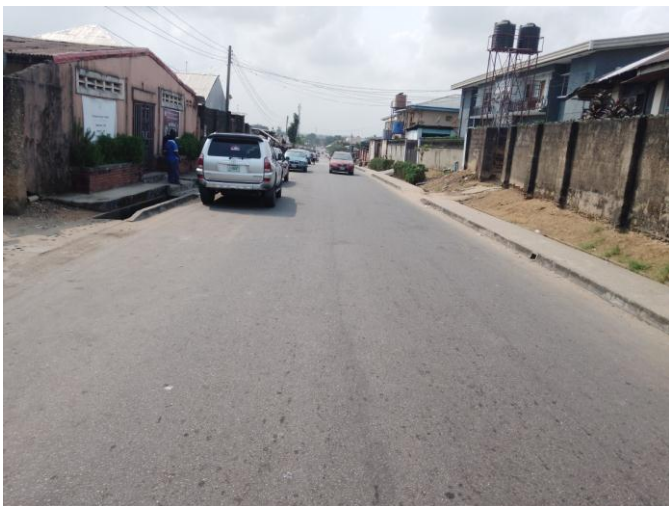
Plate 3: Webber Street by Target (Road Rehabilitation without Street Lights)
