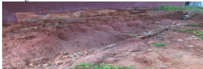
Figure 4: showing a threat to the foundation, part of school of engineering building in Auchi Polytechnic, Auchi
