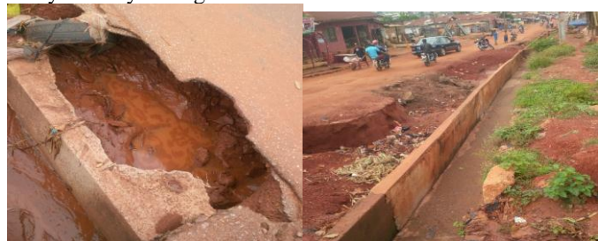
Figure 5: Gully erosion and damage to the structure along ICE road Auchi
