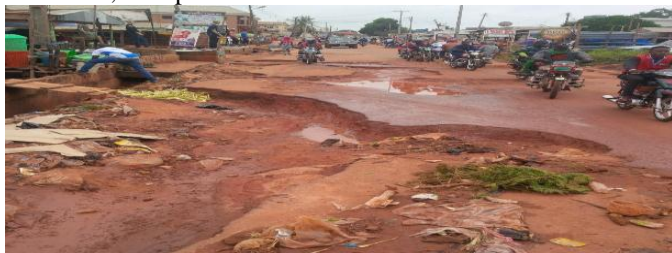
Figure 5: Gully erosion and pot holes along ICE road Auchi
