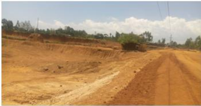
Plate 3.4: Electricity poles at Kazambeli borrow pit
