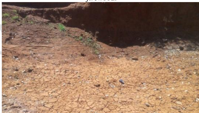
Plate 3.2: Borrow pit at Sangura as a source of water during rainy season
