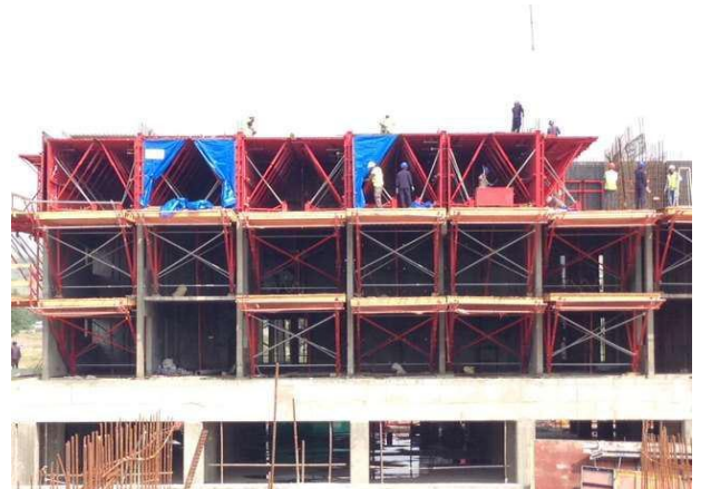
Figure 1: Tunnel formwork
