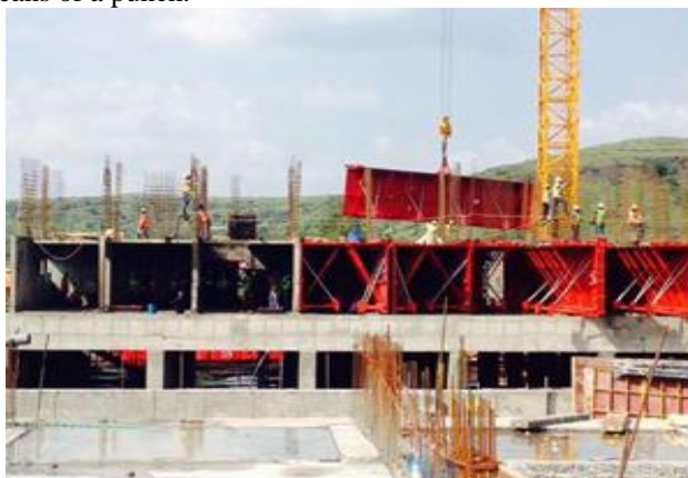
Figure 5: Stripping Of Formwork
