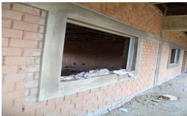
Figure 2: school building under construction
