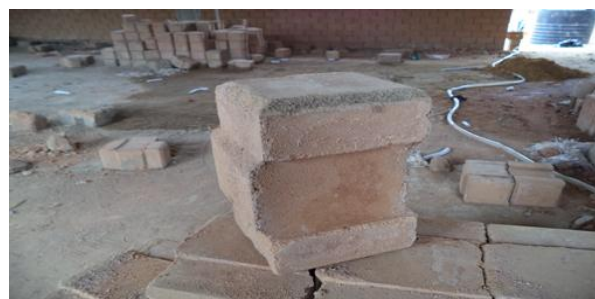
Figure 1: Interlocking soil blocks on site
