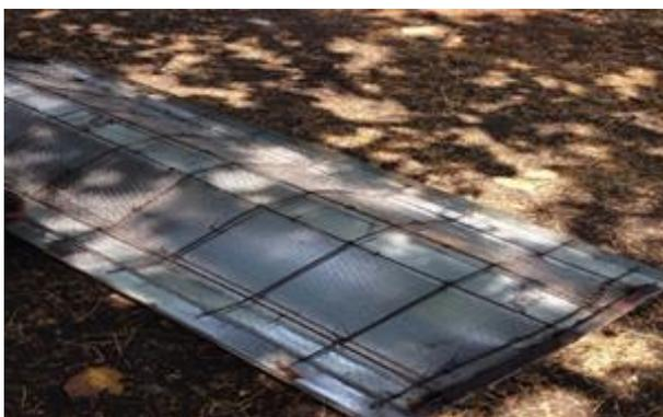
Figure 5.2: detailing of reinforcement in folded plate
