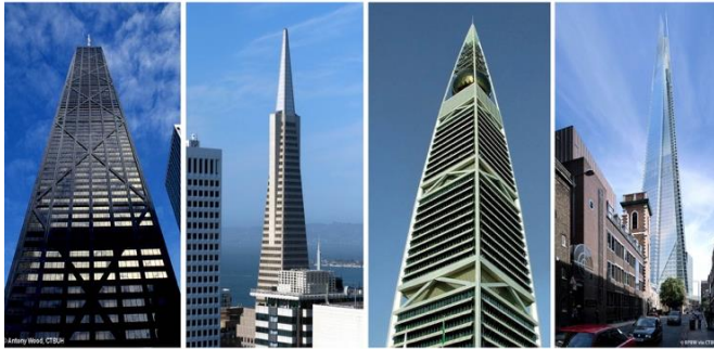
(Photo Source: CTBUH database- Skyscrapercenter.com) Figure 1: (Left-Right) John Hancock Centre in Chicago, Transamerica Pyramid in San Francisco, Al Faisaliah Center in Riyadh, The Shard in London
