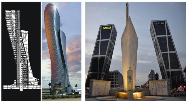
(Source: CTBUH Database-www.skyscrapercenter.com) Figure 2: (Left-Right)-Capital Gate Building in Abu Dhabi and The Gate of Europe, Madrid, Spain
