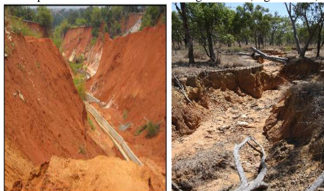
Figure 1: Typical gully site in parts of the study area
