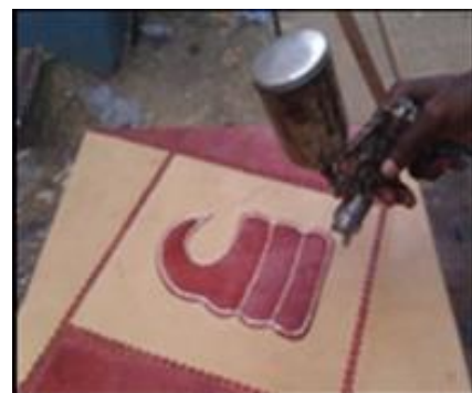
Plate 20: Spraying of tile
