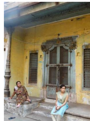
Figure 7: The typical ota space of pol house (Source: Author)
