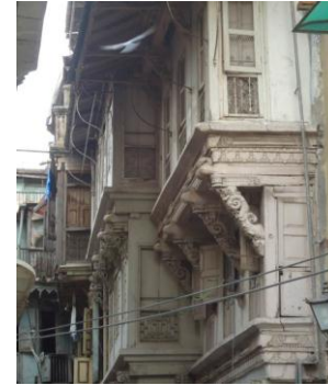
Figure 6: Brackets in pol house façade (Source: Author)
