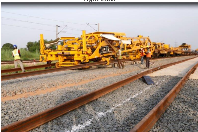
NTC track laying
