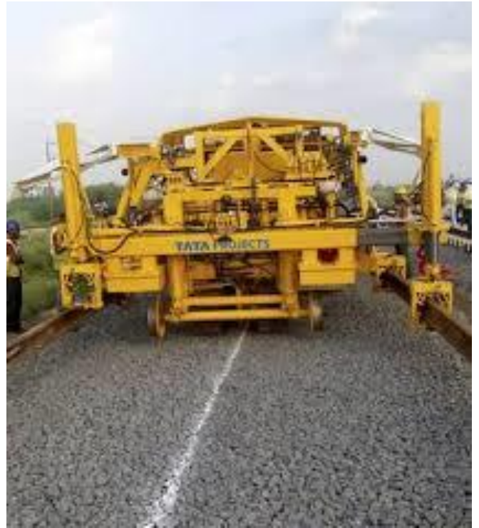
Track laying with the help of centre line
