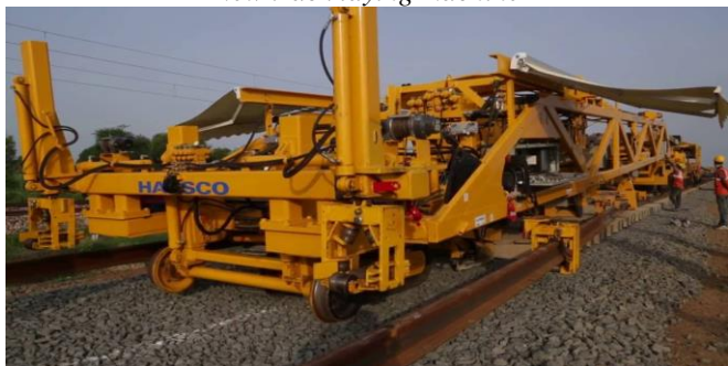
New Track Laying machine with Jupiter control system on right side.
