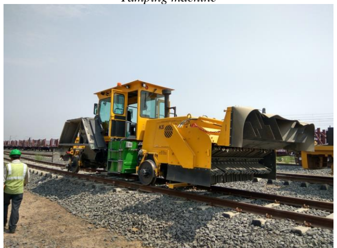
Ballast regulating machine
