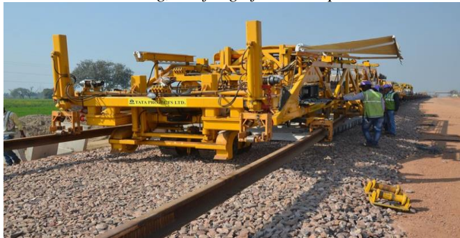
New track laying machine
