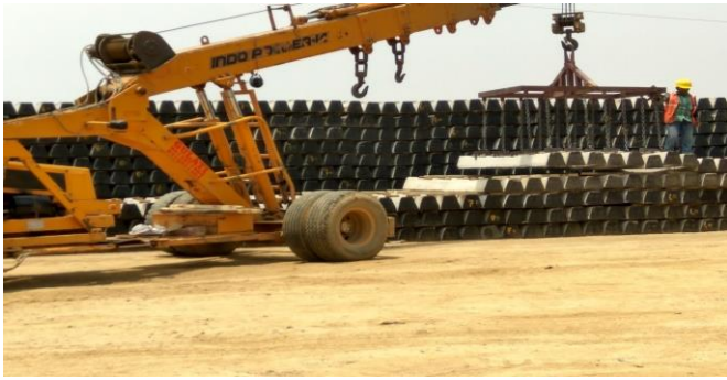
Stacking, & lifting of PSC sleepers
