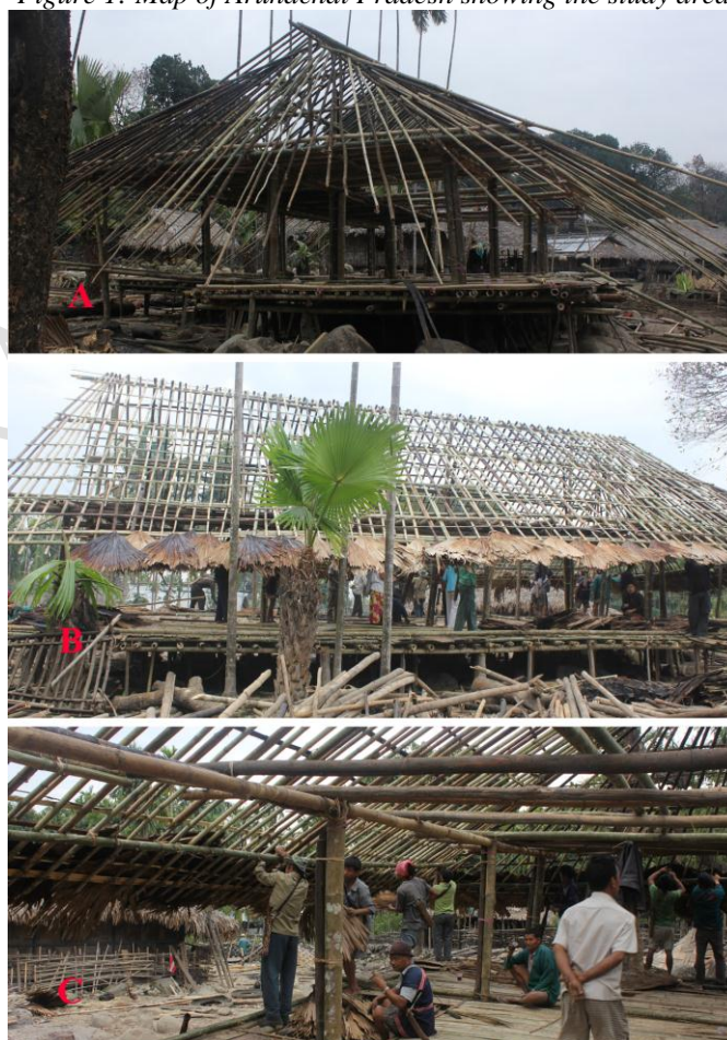
Figure 2: A. Construction in process. B & C. Thatching the complete roof frame
