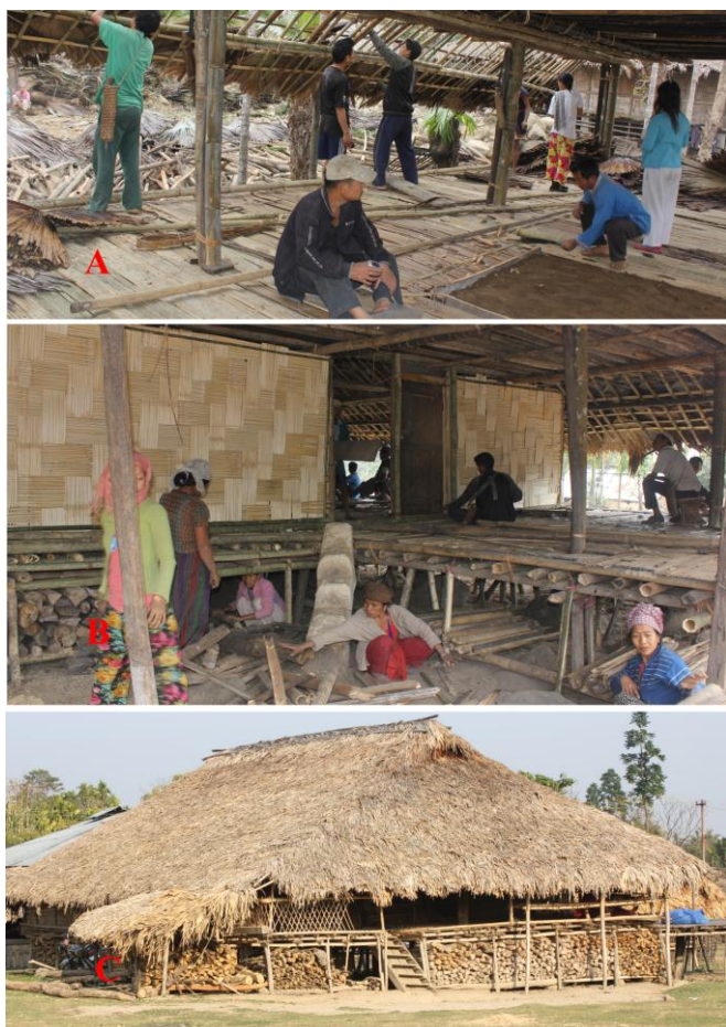
Figure 3: A. Floor made of split bamboo and fire place fill up with mud. B. The walls are made of plaited bamboo and the stilt space is used for storing firewood. C. A finished Adi house
