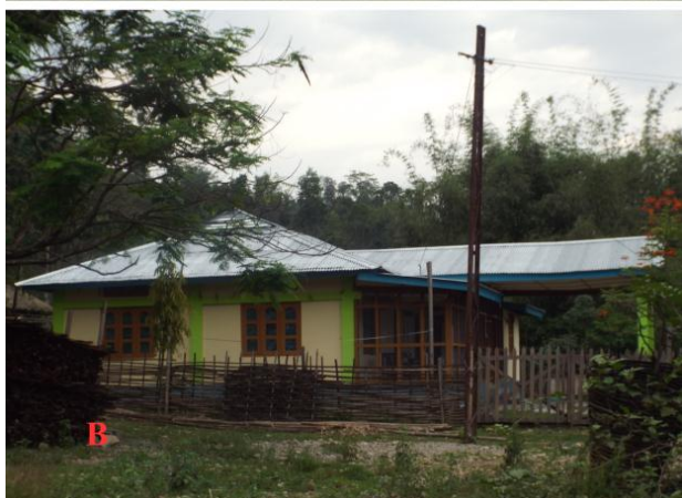
Figure 5: A & B. Windows are included in the designs; roof made of Livistona jenkinsiana leaves replaced by tin sheets; stilts made up of bamboo are replaced by concrete
